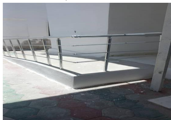
Figure 10: Renovation of Kismayo one stop center adding Front Ramps and rails for PWDs accessibility Figure 11: Renovation of Kismayo one stop center adding back Ramps and rails for PWDs accessibility
