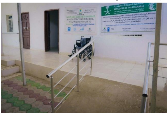
Figure 10: Renovation of Kismayo one stop center adding Front Ramps and rails for PWDs accessibility Figure 11: Renovation of Kismayo one stop center adding back Ramps and rails for PWDs accessibility
